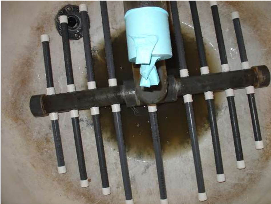
Rebuilt Lower Distributor
